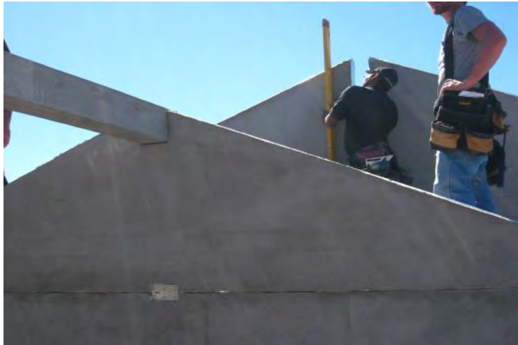
Steel and Foam Panelized construction
